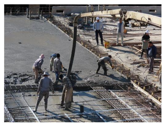
In addition, due to the significant reduction in the beam heights (about 1.2m) and the use of less concrete and reinforcement in the construction of this complex, its height and weight have also been reduced to an acceptable level compared to conventional concrete methods, which had also increased the structural resistance against earthquakes.
