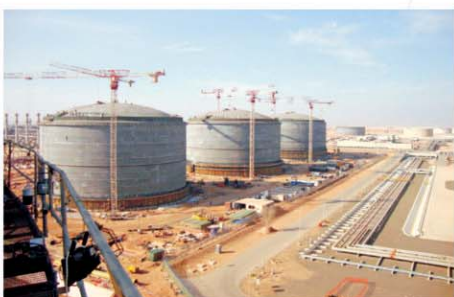
Post Tensioned Reservoirs
