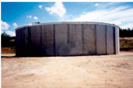
5ML East Bowral Reservoir hidden within the wall
