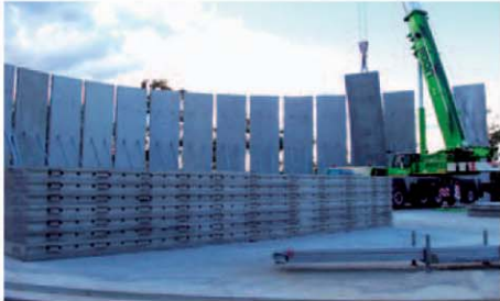
Pre-cast wall being erected
